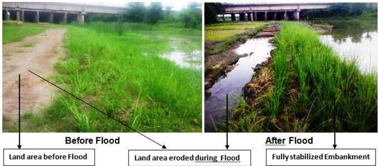
Stabilized River Embankment
