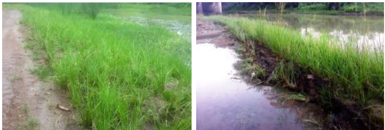
River Embankment Stabilization & Restoration through Bio-engineering techniques
